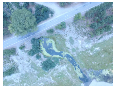
Figure 7. In the image, you can see the river called Karchaghbyur, which empties into Lake Sevan and is one of the sources of the lake's water pollution. As could be seen in the image, algal blooms are a direct indication of increased flux of nutrients into the lake. Satellite and drone images are great tools to identify such sources in vast surface areas. This image is representative of the whole Black Sea Basin as currently, the rivers are one of the greatest sources of Black Sea pollution.
